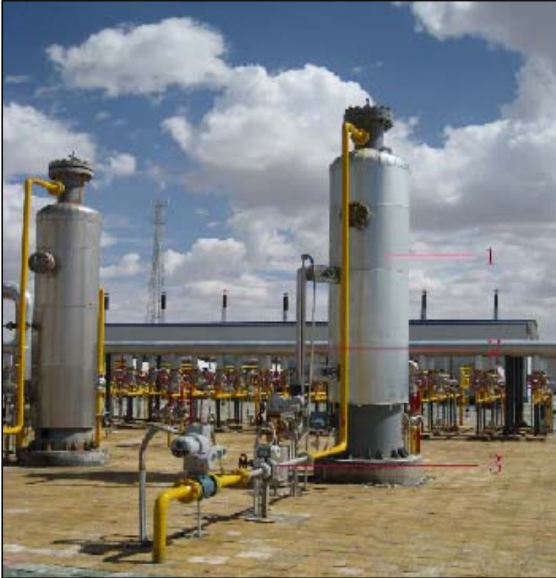
Figure 3 - Conventional Test Setup at the SeBai gas well
